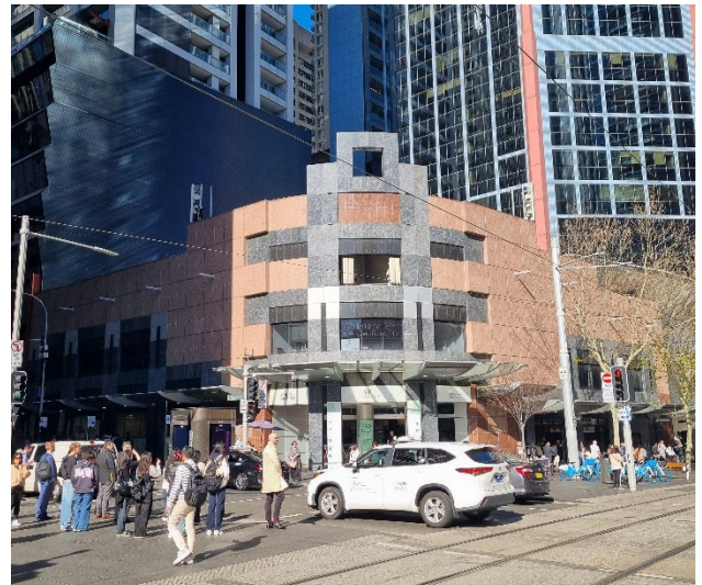
Picture 2 View of Site from George Street and Bathurst Street Intersection (close)
